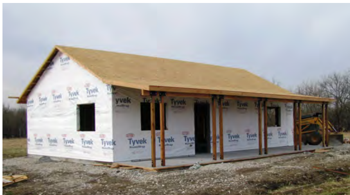
Construction of KDWPT headquarters is expected to be completed by June.
