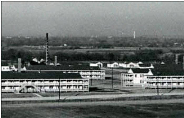
H-shaped dormitories were located just to the east of the former administration building.
