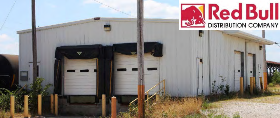
Building 1629 at Great Plains Industrial Park is the new home of Red Bull Distribution Company.
