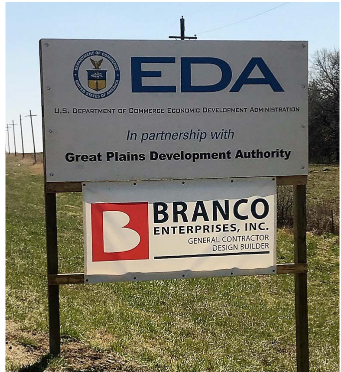
A newly erected sign at the industrial park informs tenants and visitors of the EDA funded project currently underway.
